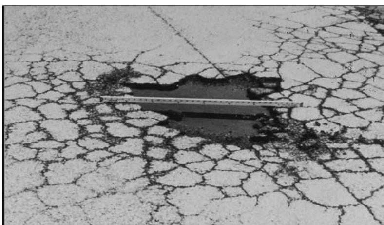
FIGURA 63: Severidad Alto (H) de Parches. FUENTE: American society for testing and materials, 2018.
