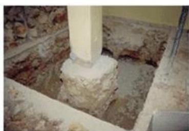
Fig.1: Excavation around the footing
