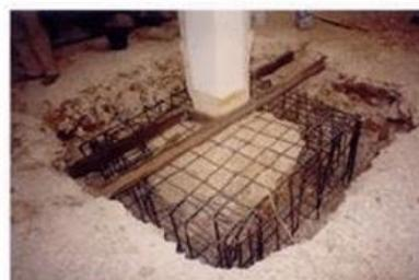
Fig.4: Completing the jacketing of footing
