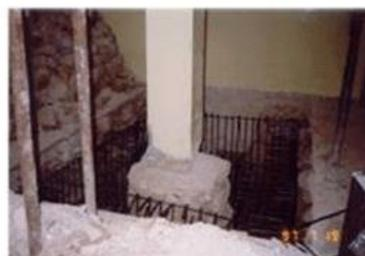
Fig.2: Hardening the surface and installing dowels in footing
