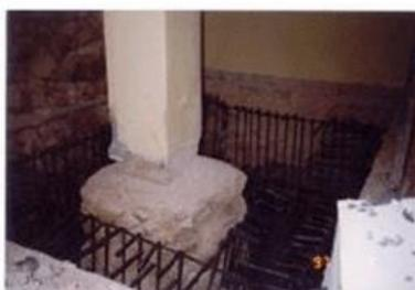
Fig.3: Installing the main steel in
