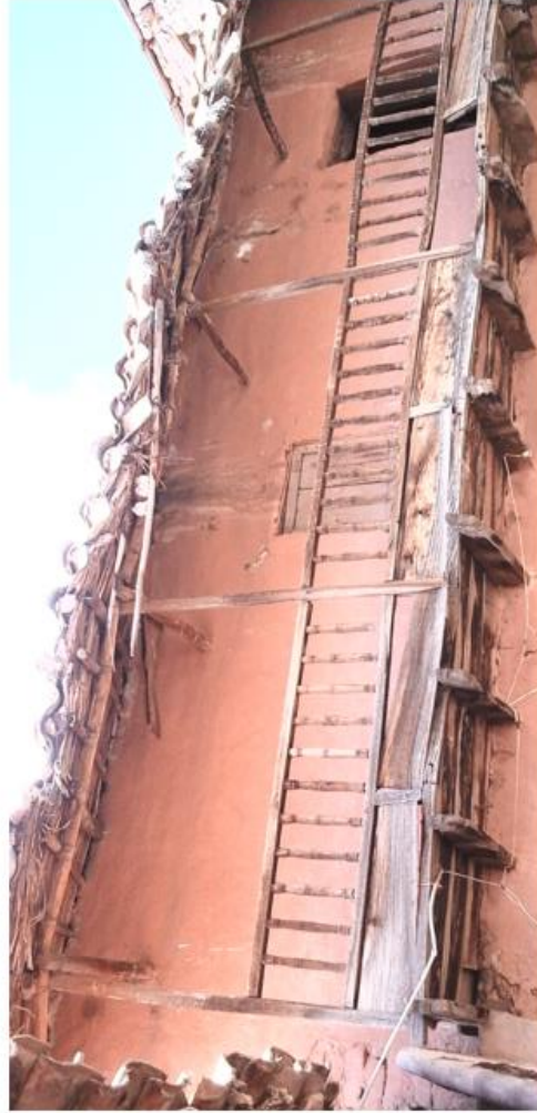
Vista de Balcón interior
