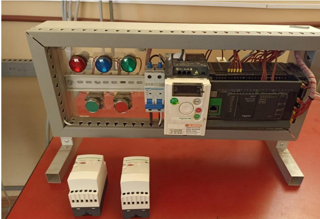
**Figura 13:** PLC Modicon, modelo M241, Schneider Electric
