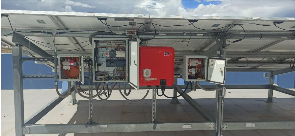
Figure 10 Installation of the SFCR String data acquisition system.
