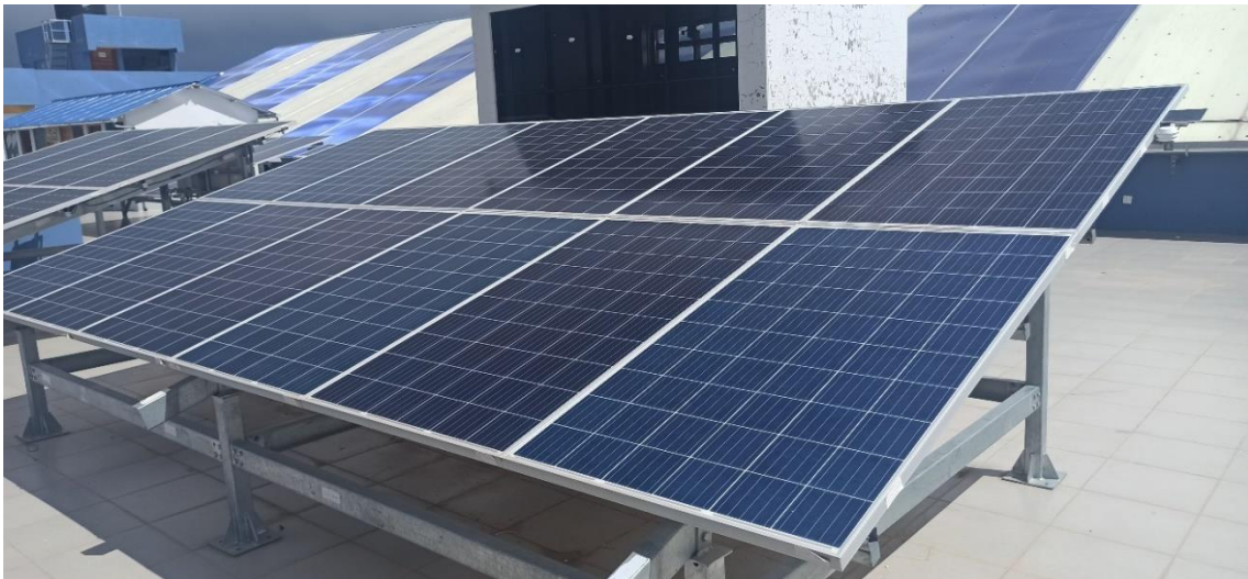
Figure 5 SFCR installation with String inverter.
