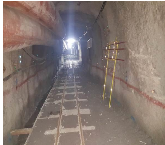
By Pass Túnel 4
