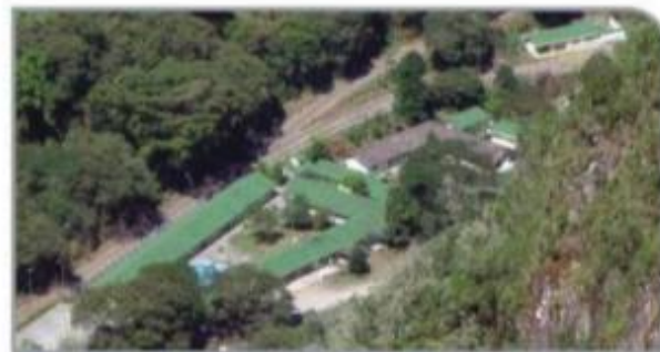
CENTRAL HIDROELECTRICA - CUSCO
